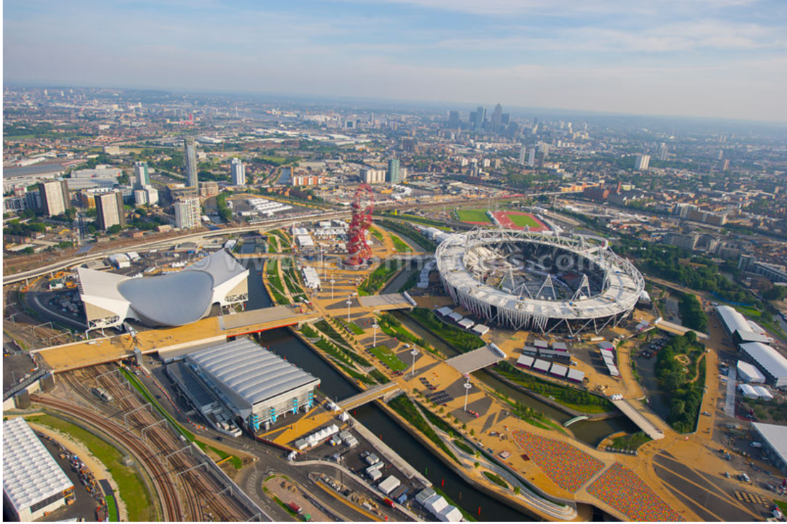
Olympic Stadium, London, United Kingdom
