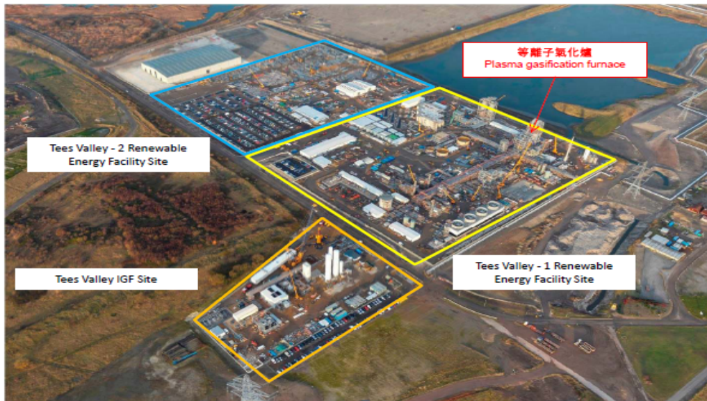
Aerial view of Air Products' waste-to-energy facilities in Teesside
