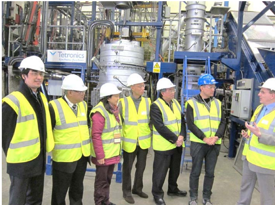
Members of the delegation received a briefing on the operation of APP's pilot plasma gasification plant
