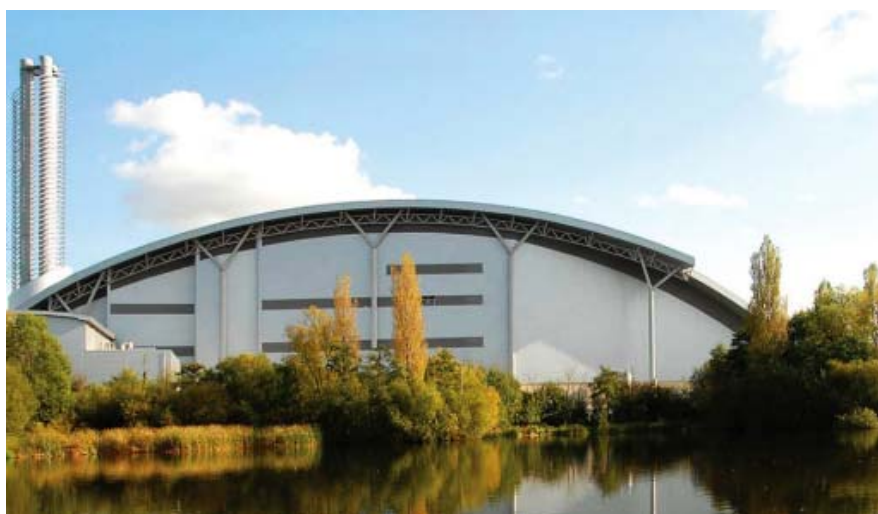
Lakeside Energy-from-Waste Plant
