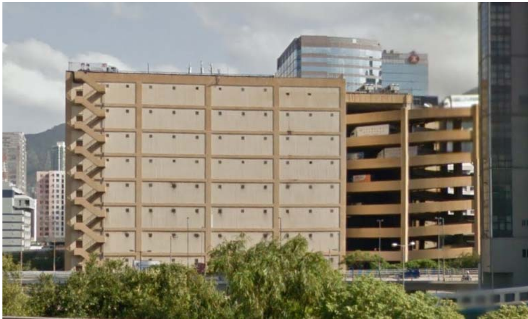
Figure 5 An existing multi-storey cargo centre in Kowloon Bay
