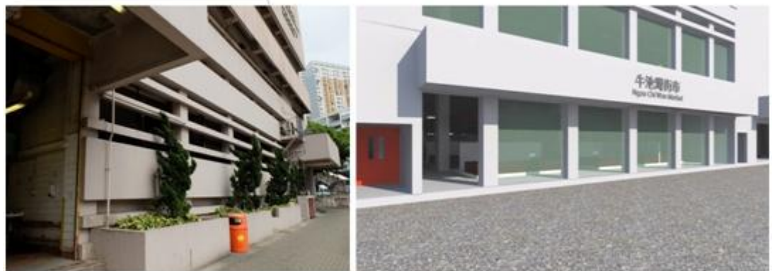
Facade facing Lung Cheung Road
