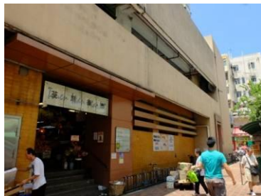
Market façade not distinctive
