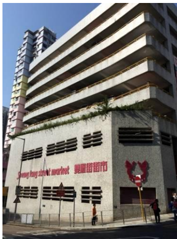
Market façade not distinctive
