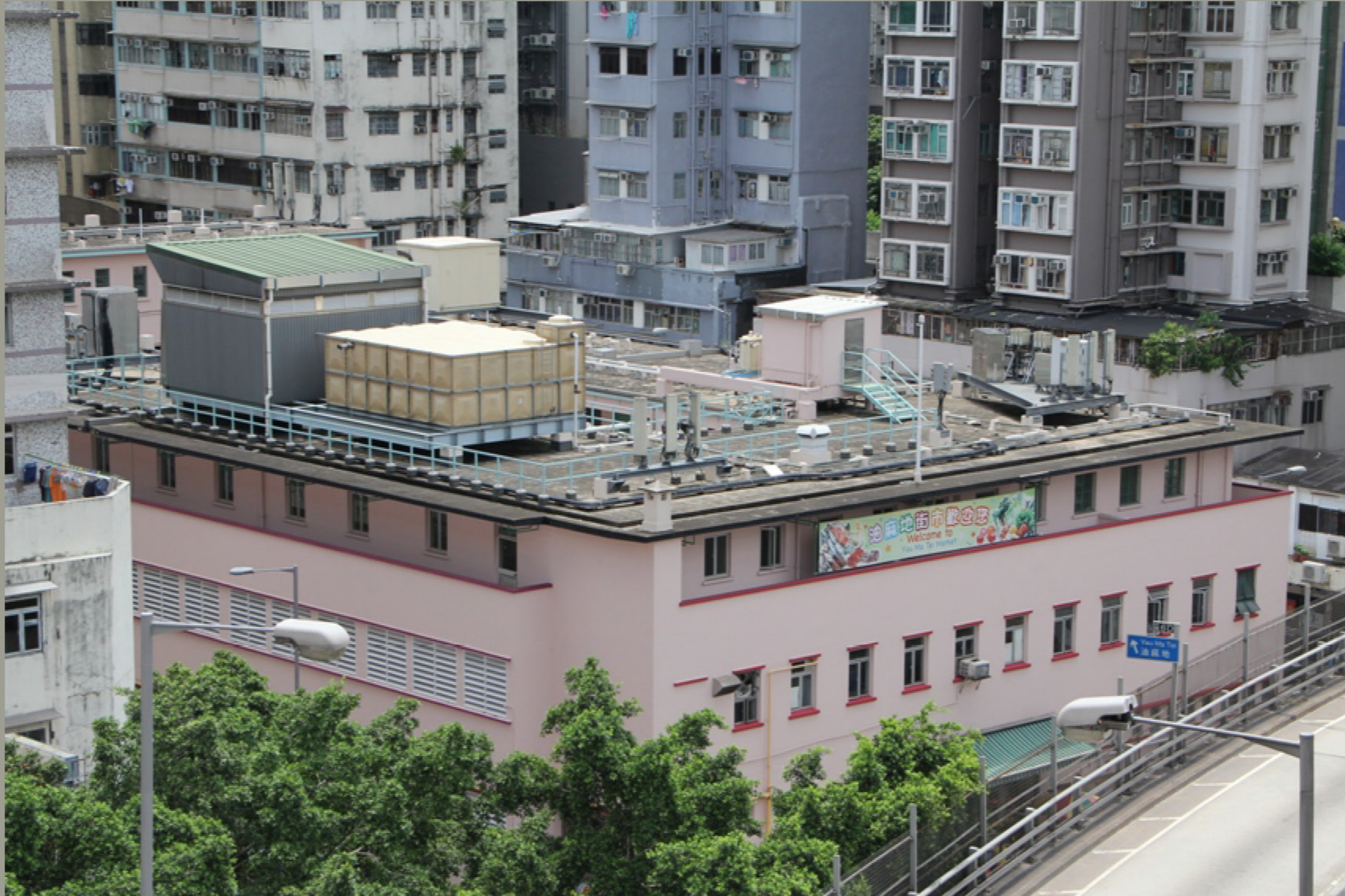
EXISTING STRUCTURE ON ROOFTOP
