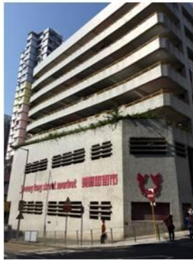
Sheung Fung Street Market façade. The two-floor market is located below a public car park.
