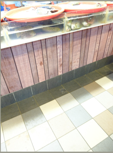
Only a small floor drain along aisle
