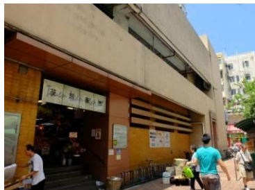
Market façade not distinctive
