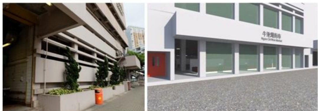
Facade facing Lung Cheung Road
