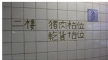
TENANTS MADE THEIR OWN NOTICES
