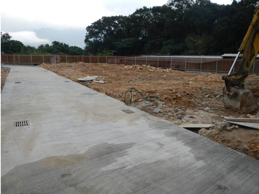
Figure 7. The so-called ‘farm’, seems to be ‘under construction’
