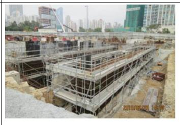
WKT Excavation underneath B3 slab at north top down area (810A) Phase 3 blasting laying hanging mat (810A) Blasting under preparation (810A)
