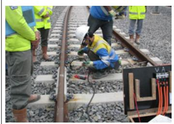
Overhead Line Continuity and Insulation Pre-test at Restricted Area (830)
