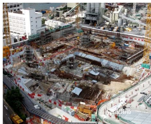
Works on site (June 2015)
