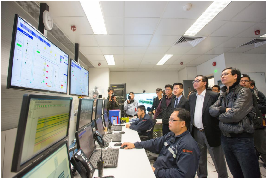
Legislative Council Members observe the control room of the northern plant of the district cooling system at the Kai Tak Development.
