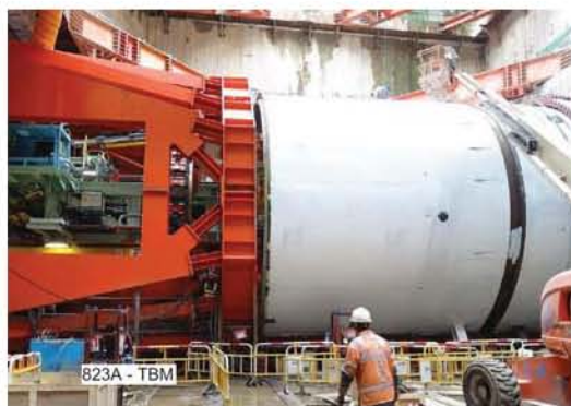
TBM at contract 823A
