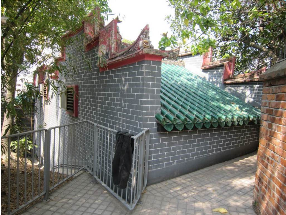
The stepped gables of the rear hall in the style of “五岳朝天” (which literally means “five peaks paying tribute to heaven”)
