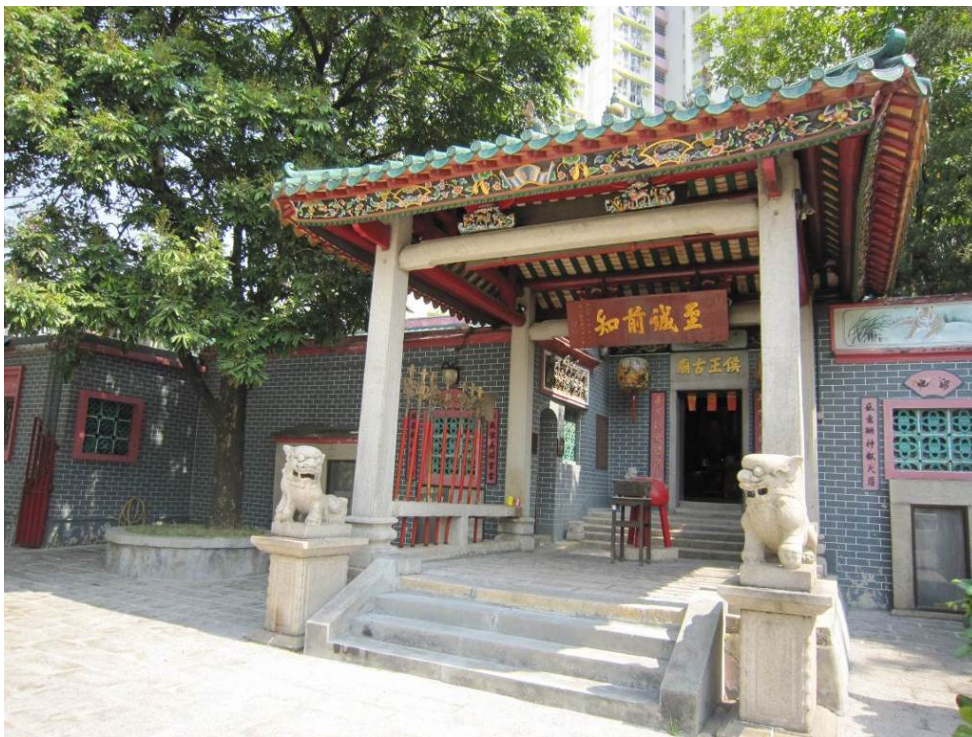
A detached pavilion with hip-and-gable roof in front of the main temple building
