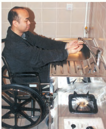
Under universal design for MFD, the sinktop inside the kitchen of a modular flat can be placed at a convenient height for wheelchair users.
