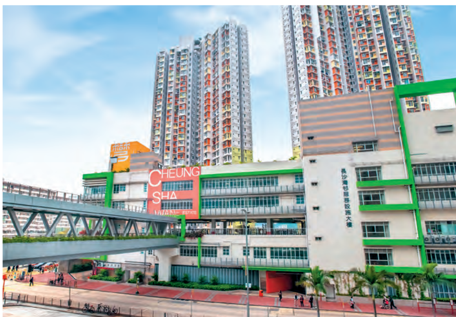
Ancillary Facilities Block, Cheung Sha Wan Estate.
