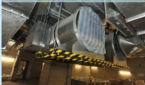
環控系統風扇 Fans of Environment Control System
