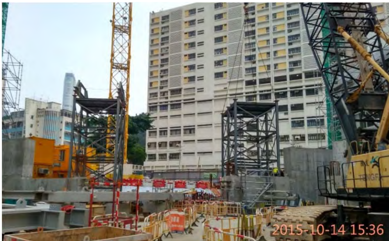
Mega Truss 5 assembled 5 號主要支架組裝
