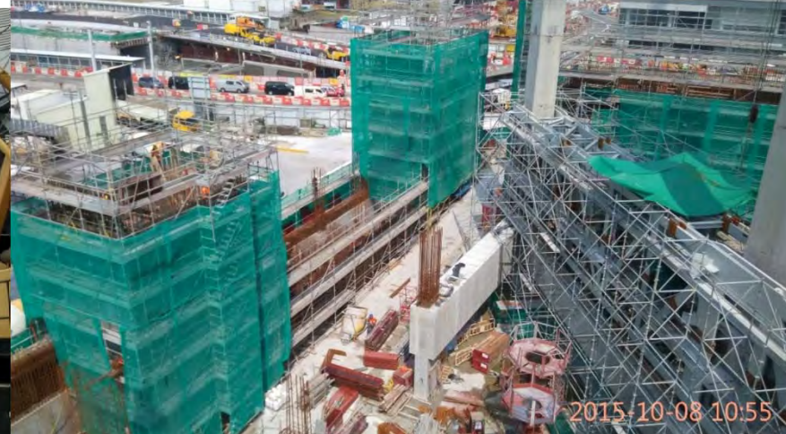
Construction of core walls to 2 nd Floor 主力牆已興建到2樓
