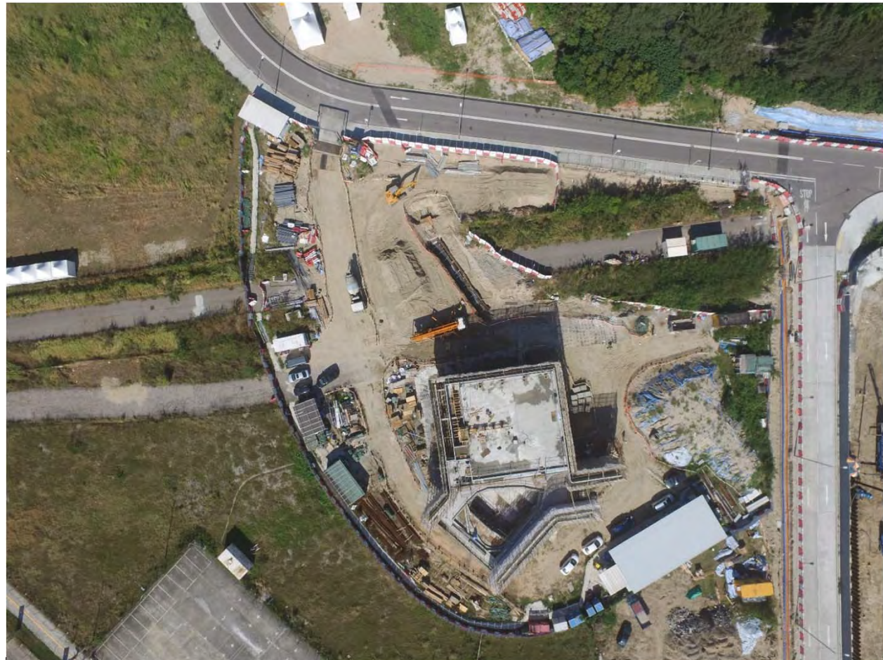
Construction of Building Structure and External Underground Utilities
