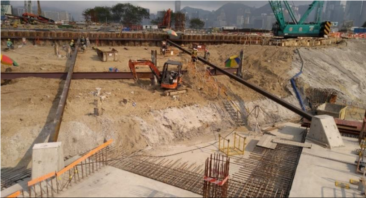
Phase 2 Excavation and Lateral Support (ELS) Works 第二階段挖掘工程側向支撐安裝
