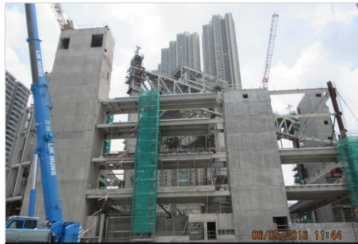
Perimeter Steelwork (West Elevation) and Slab Construction 外圍主要鋼結構支架(西面)及樓板安裝
