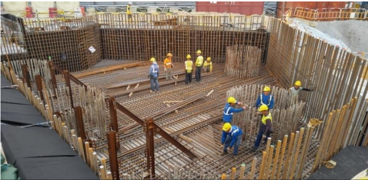
Reinforcement Fixing for Pile Caps 樁帽鋼筋固定工作
