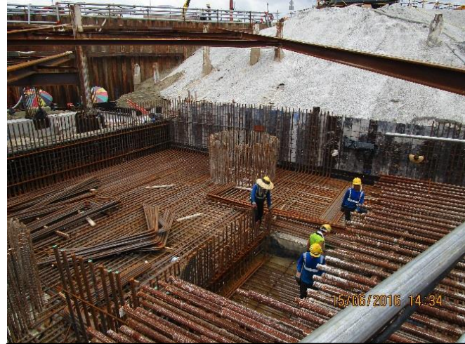
Rebar Fixing for Pile Cap 固定樁帽鋼筋
