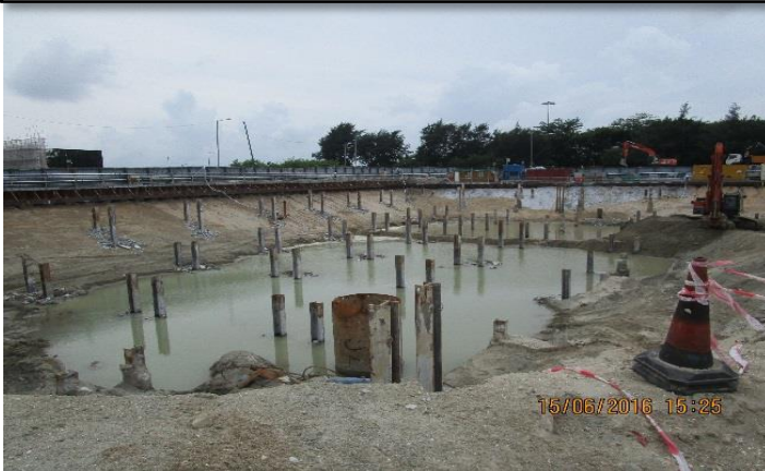
Excavation Works for Interfacing Car Park Area 地庫停車場挖掘工程
