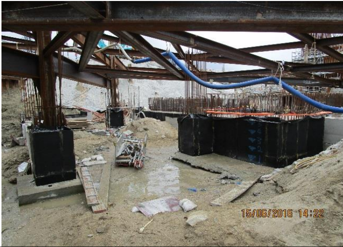
Excavation and Lateral Support (ELS) Works 挖掘及側向支撐安裝工程
