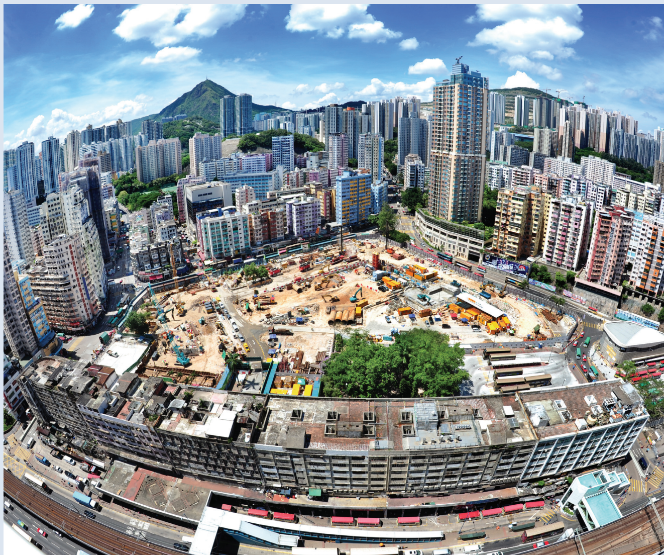
■ Panoramic overview of Kwun Tong Town Centre project site.
