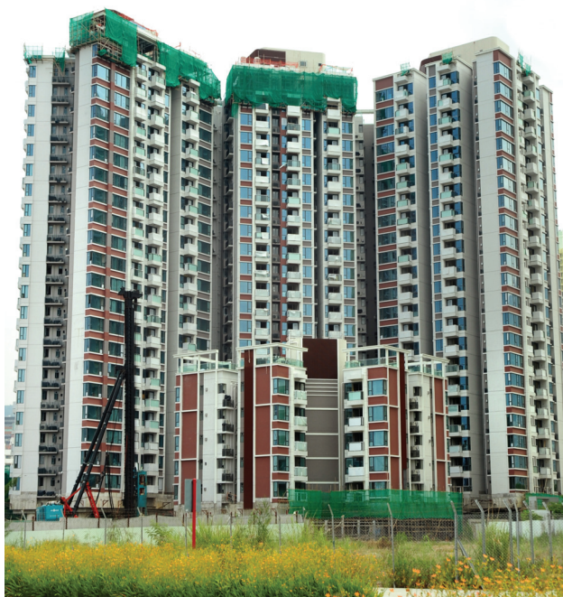
Existing view of De Novo.
