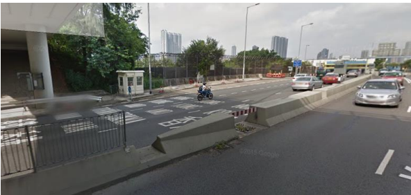
Unprotected kiosk for operational staff and hazardous discontinuity of the median barrier.
