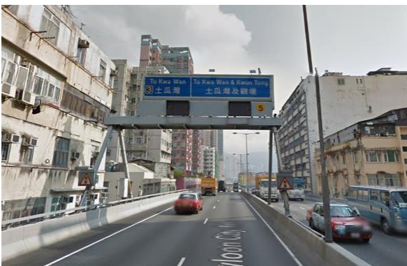
Contrary to the sign display, right lane traffic cannot access "To Kwa Wan" whereas left lane traffic can also access "Kwun Tong". Information on the upstream sign is also inconsistent with that on the downstream sign. Misleading signage on high speed roads is a significant safety problem.
