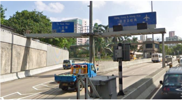
Guidance to "To Kwa Wan" on westbound tunnel tube is too late. Advance direction signs for the exit are missing.
