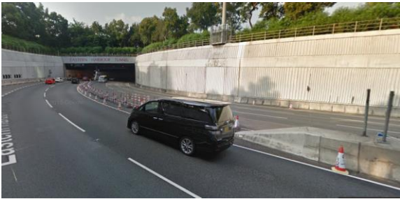
The median opening at the Quarry Bay tunnel entrance entails the risk of head-on collision if a vehicle loses control on the tight bend.
