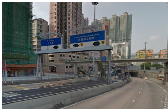
Contrary to the sign display, right lane traffic cannot access "To Kwa Wan" whereas left lane traffic can also access "Kwun Tong". Information on the upstream sign is also inconsistent with that on the downstream sign. Misleading signage on high speed roads is a significant safety problem.
