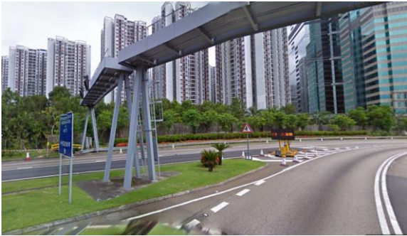
Unguarded support posts for traffic control system equipment are safety hazards.
