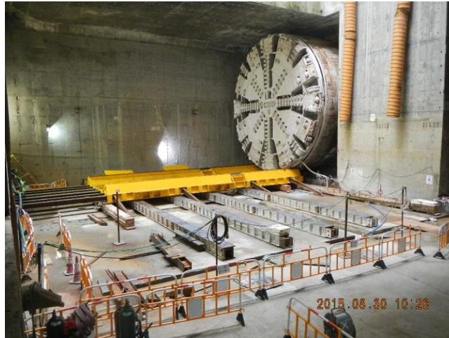
Tunnel breakthrough of northbound track tunnel of Contract 826
