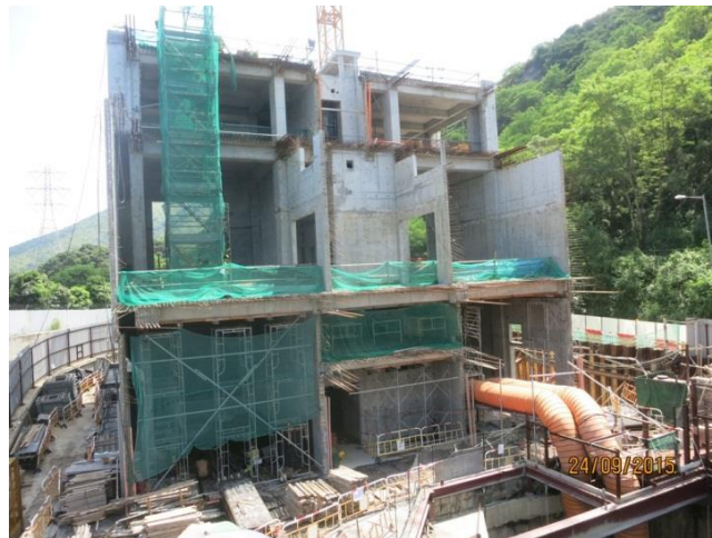
Overview of Ngau Tam Mei Ventilation Building
