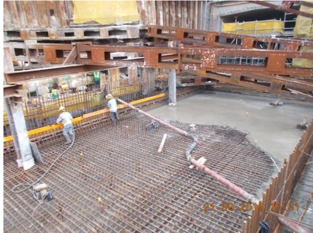
Concreting of Lin Cheung Road Underpass slab
