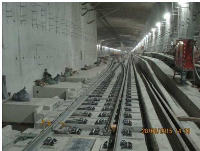
Overhead line installation and track-laying works inside the tunnels
