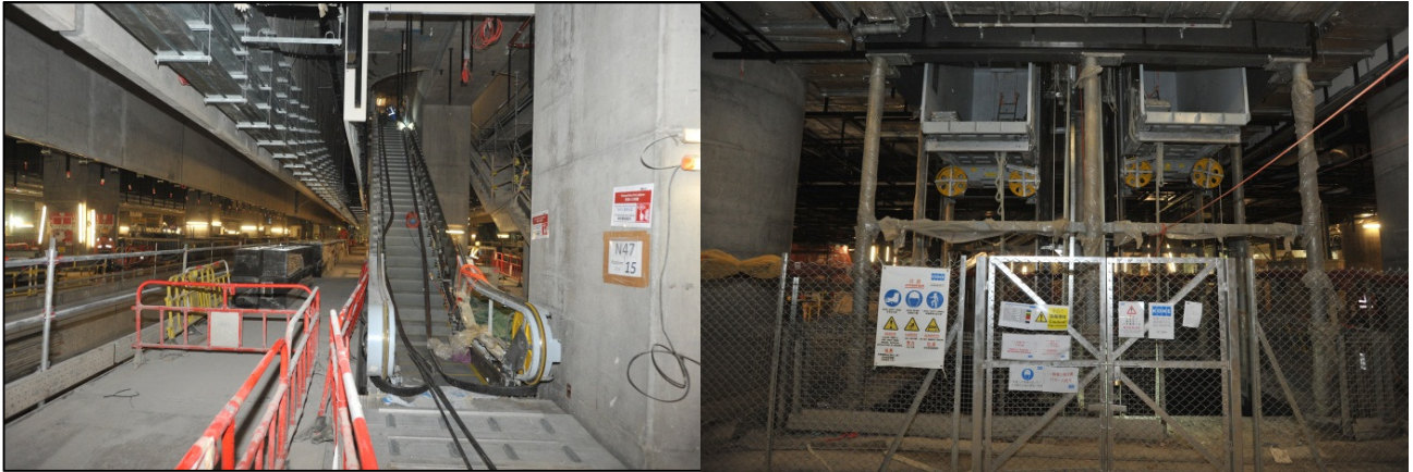
Installation of escalators and lifts at WKT is in progress
