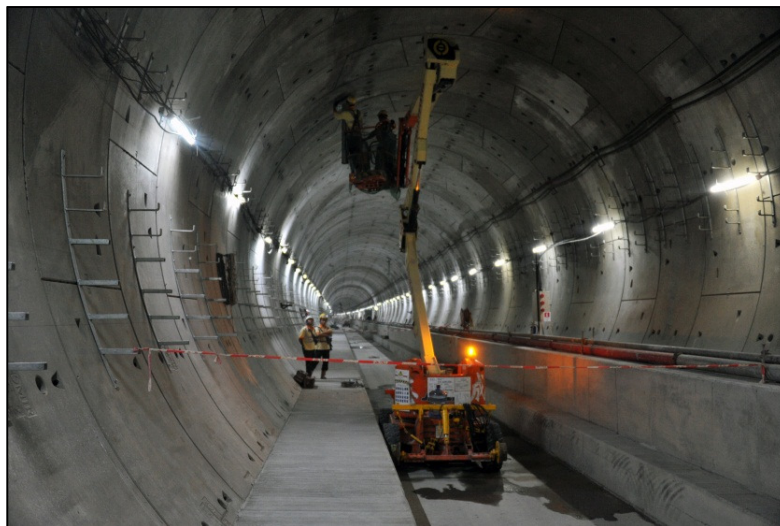
Installation of overhead lines along the tunnel section
