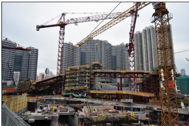
V-Trusses erection in progress at WKT
