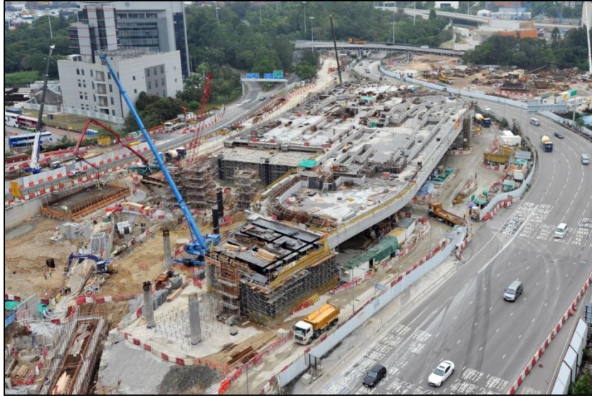
Construction of the new PTI landscape deck
