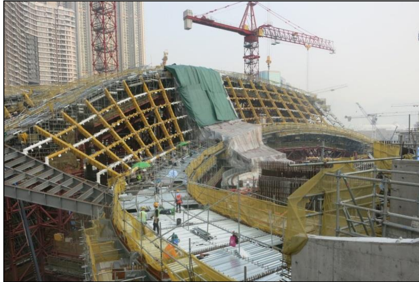
V-Trusses erection in progress at WKT
