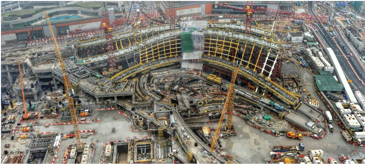
Structural works for Station Entrance Building at WKT
