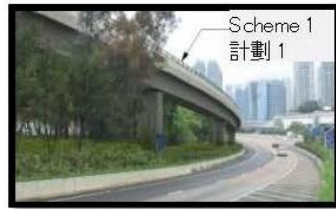
Scheme 1 計劃 1 Proposed single lane elevated road connecting Hoi Po Road to West Kowloon Highway northbound 擬建高架單線行車道連接海寶路至西九龍公路北行方向
