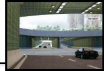
Depressed Austin Road West and Lin Cheung Road junction 低於地面的柯士甸道西與連翔道交匯處
