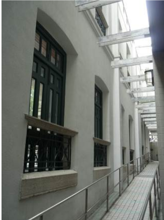
View behind the façade showing the inner skin of the old wall on the left, with the original window openings still intact.
