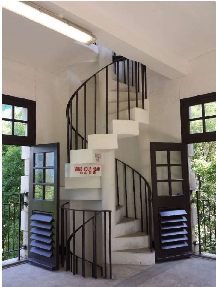
Concrete and steel spiral staircase on 1/F
