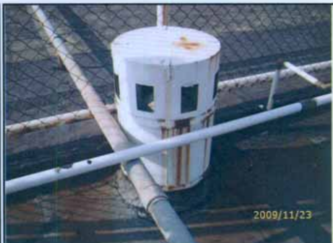
2. DESCRIPTION : Encapsulated ACM refuse chute at roof floor
