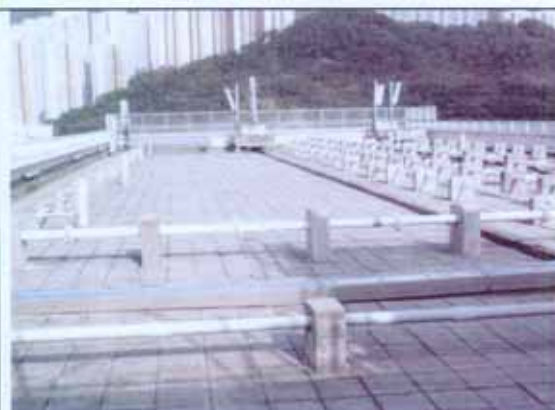
Vent pipes At roof
