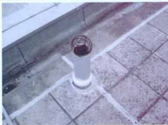
Vent pipes at roof
