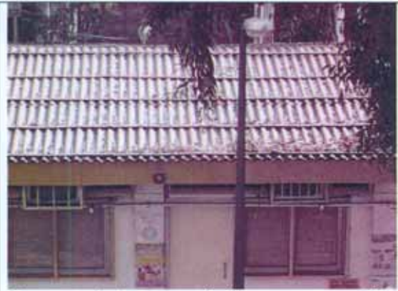
Corrugated sheet at roof of management office
