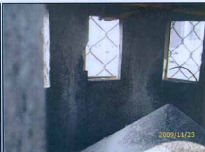
4. DESCRIPTION : ACM refuse chute at roof floor
