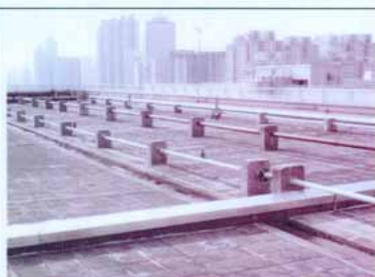
Vent pipes at roof
