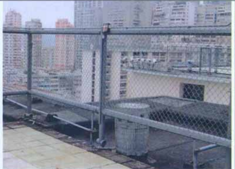
Refuse vent pipe at roof
