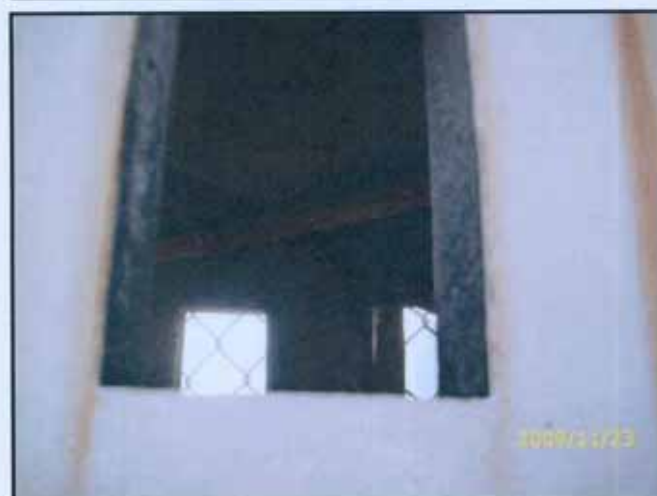
5. DESCRIPTION : ACM refuse chute at roof floor
