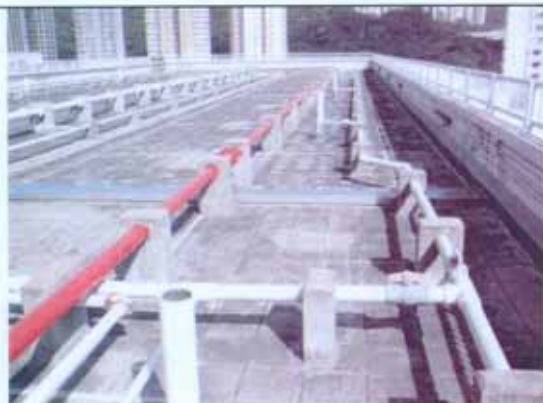
Vent pipes at roof
