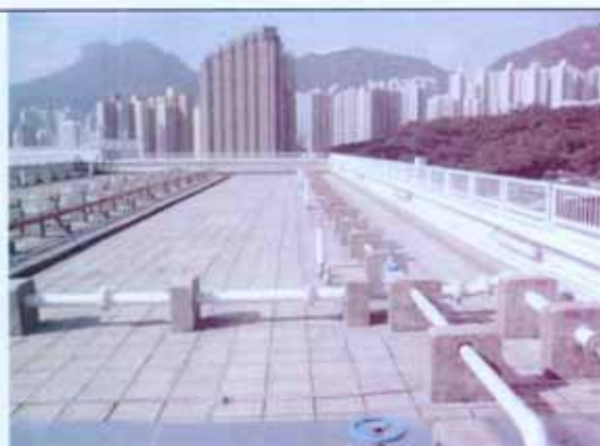
Vent pipes at roof
