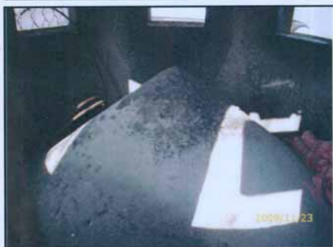
3. DESCRIPTION : ACM refuse chute at roof floor
