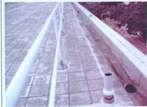
Vent pipes at roof
