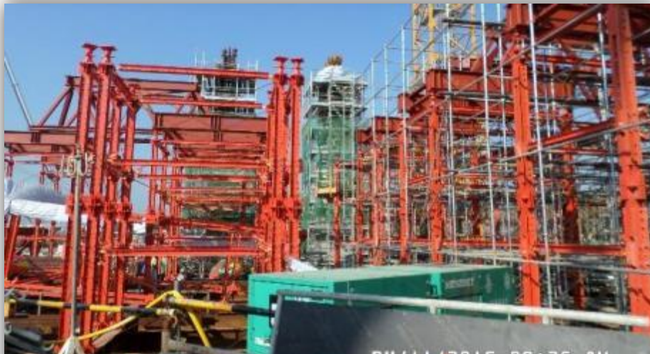
Falsework for truss T1 and T2 installation T1及T2 安裝工程
