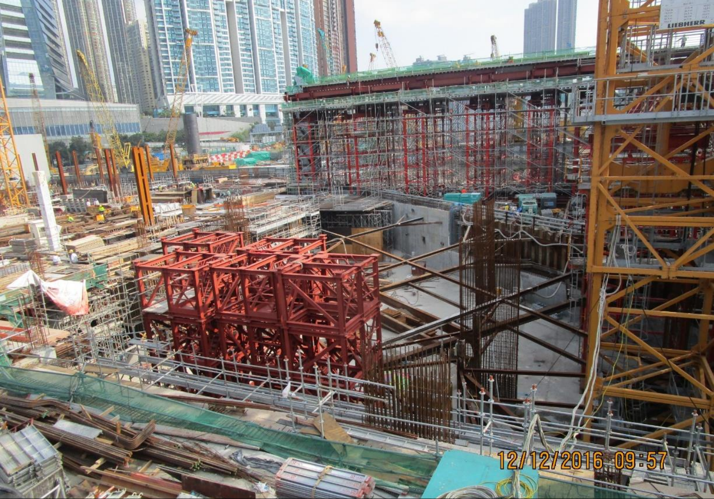
Temporary Supporting Towers for Truss 5
