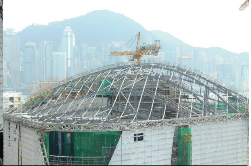
Roof Structure completed 頂部結構已完成
