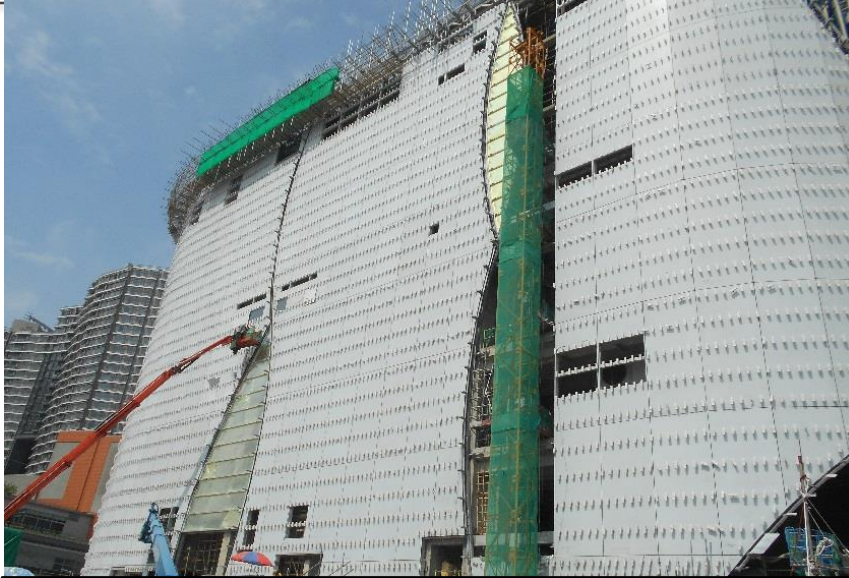
Façade installation at west elevation 安裝西面外牆
