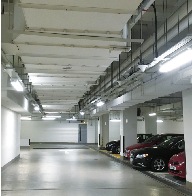
Fluorescent lights at Bio-Informatics Centre car park were replaced by motion/photo sensor-embedded LED lights to save energy
