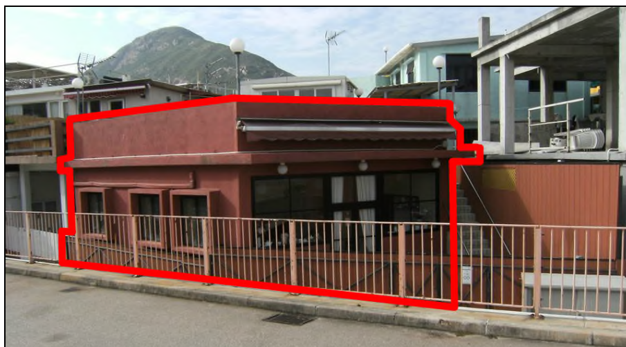
SS Structure B (December 2016)
