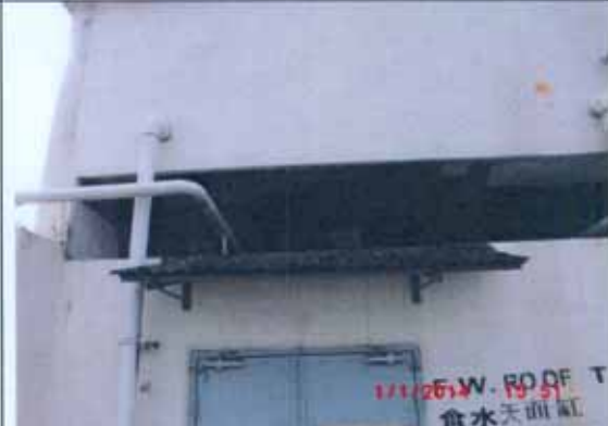
Corrugated sheet below water tank at roof
