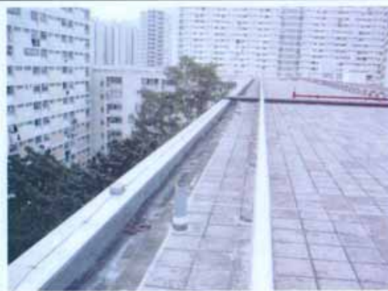
Vent pipes at roof
