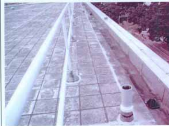
Vent pipes at roof
