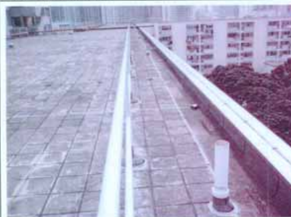
Vent pipes at roof
