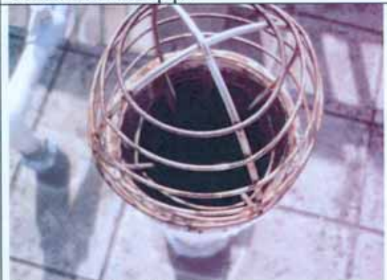
Closed up view of vent pipe
