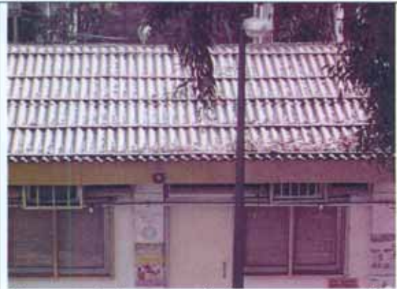
Corrugated sheet at roof of management office
