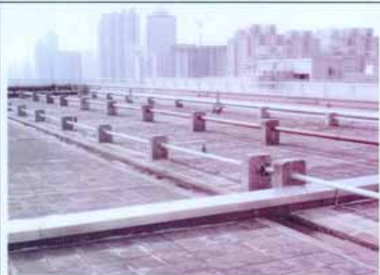
Vent pipes at roof
