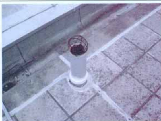
Vent pipes at roof
