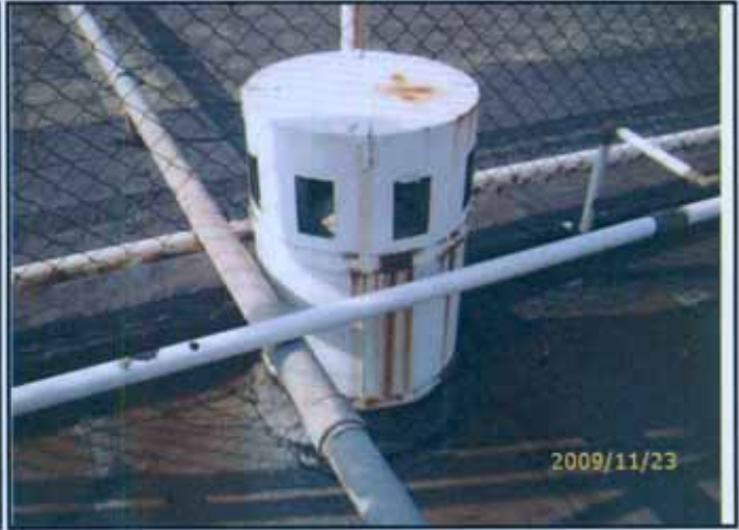
2. DESCRIPTION : Encapsulated ACM refuse chute at roof floor
