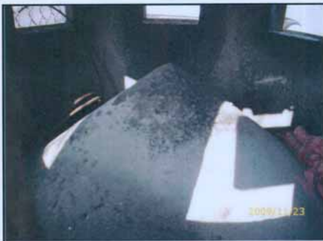
3. DESCRIPTION : ACM refuse chute at roof floor
