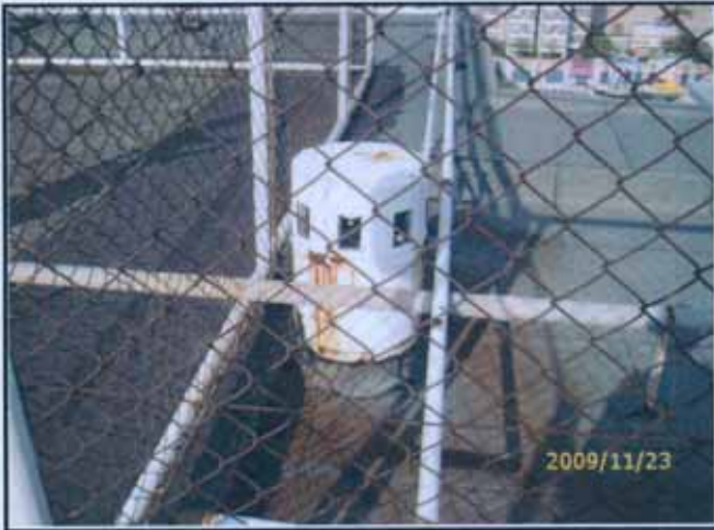
1. DESCRIPTION : Encapsulated ACM refuse chute at roof floor
