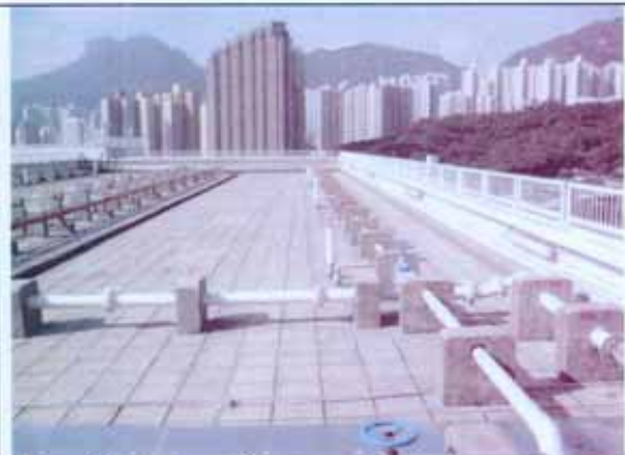
Vent pipes at roof
