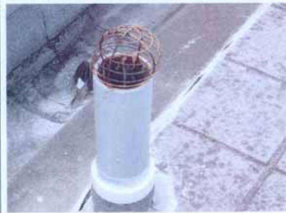
Vent pipes at roof
