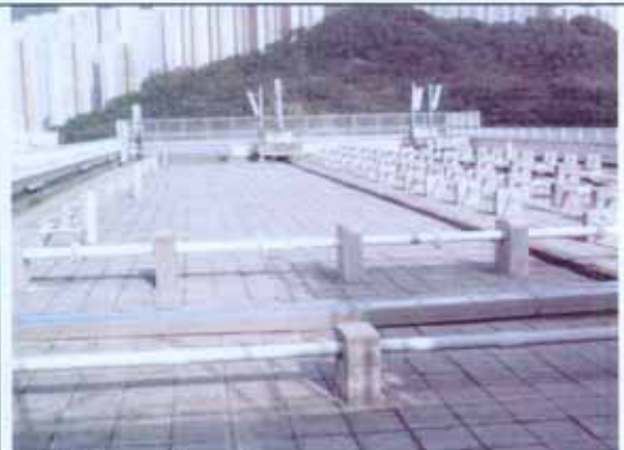
Vent pipes At roof
