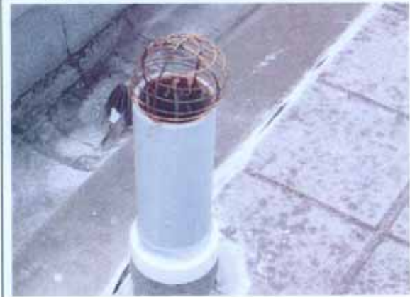
Vent pipes at roof
