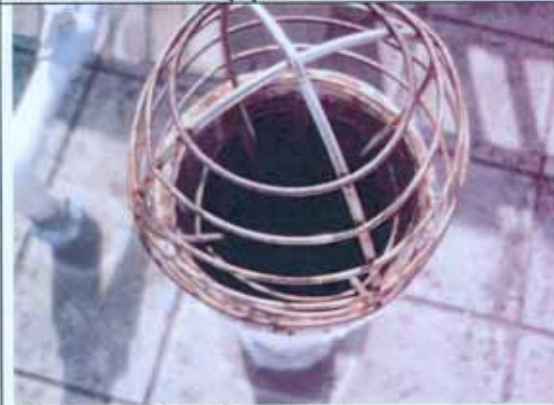
Closed up view of vent pipe
