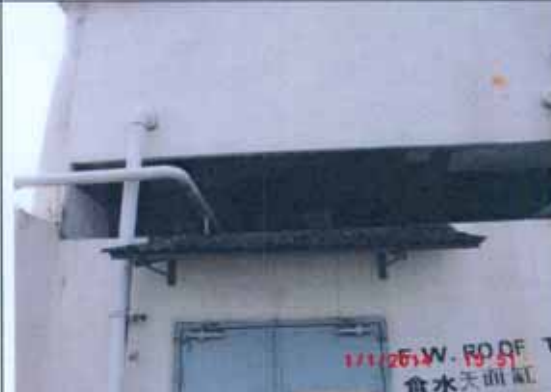
Corrugated sheet below water tank at roof
