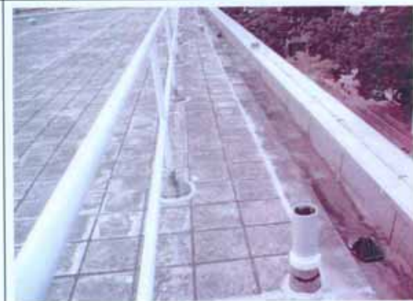
Vent pipes at roof
