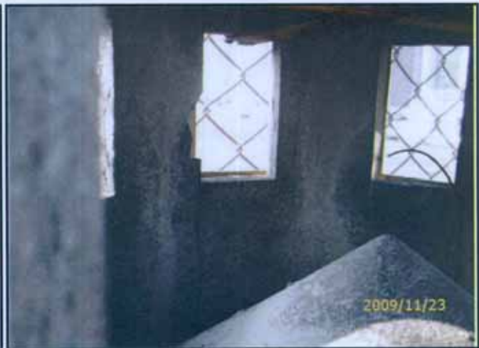
4. DESCRIPTION : ACM refuse chute at roof floor
