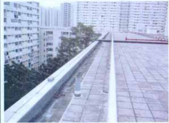
Vent pipes at roof
