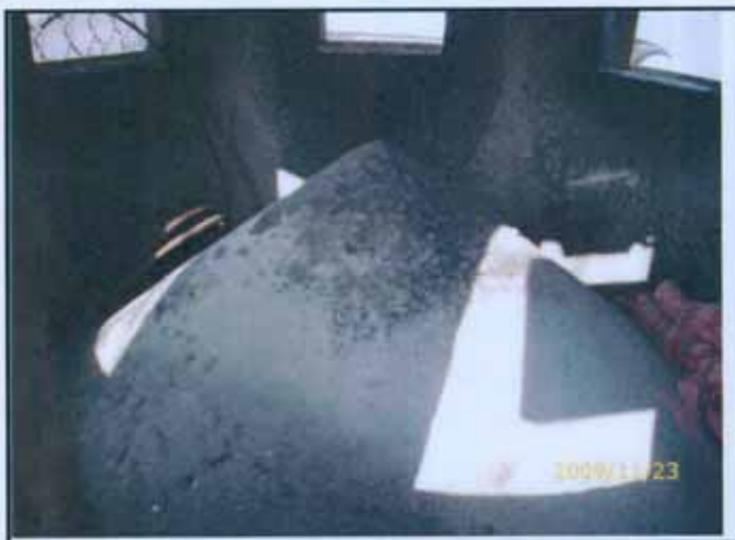
3. DESCRIPTION : ACM refuse chute at roof floor
