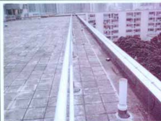
Vent pipes at roof
