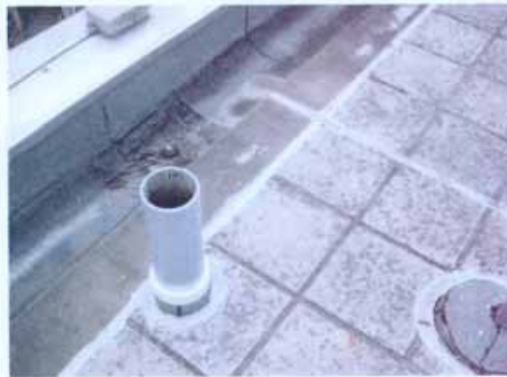
Vent pipes at roof
