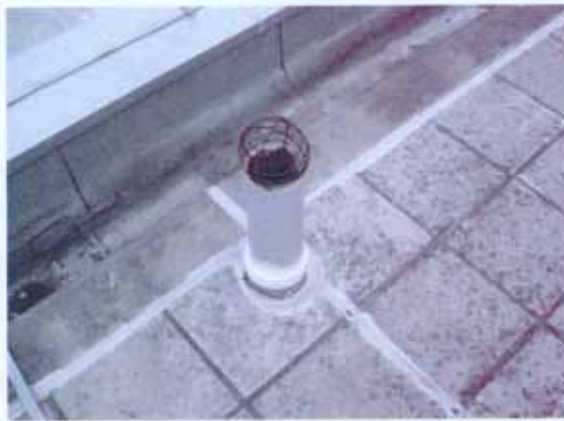
Vent pipes at roof
