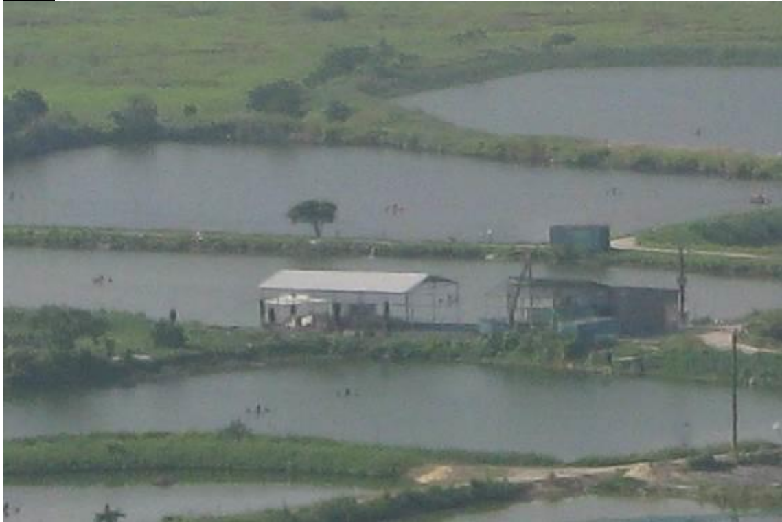
Fig 5c The emergent structure remains in the pond, only the roof that encroached into the Government land has been removed (photo taken on 19 June 2015)
