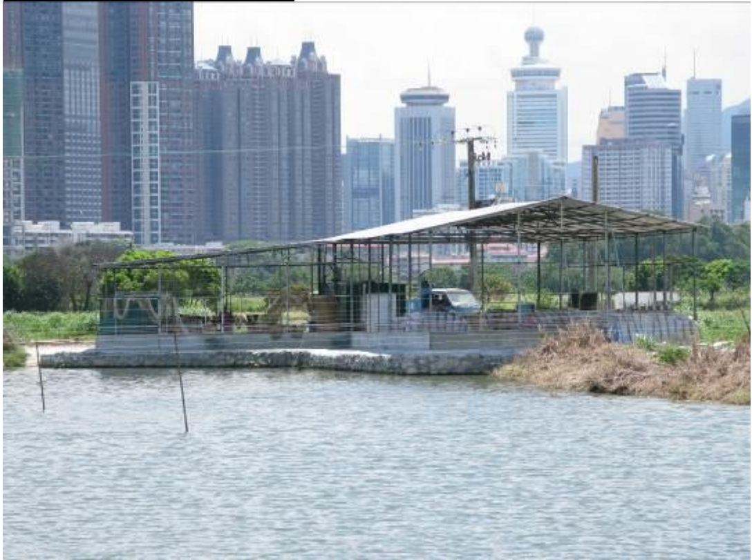
Fig 5a Unauthorised development in the E/NE-MTL/003 case at Hoo Hok Wai (photo taken on 19 June 2015)
