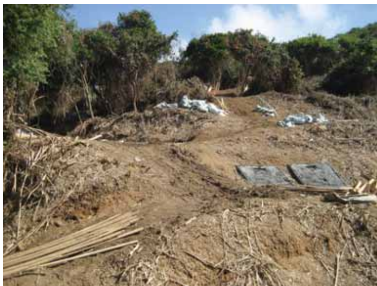
Suspected site formation and vegetation clearance on Po Toi Island. © Geoff Welch/HKBWS
