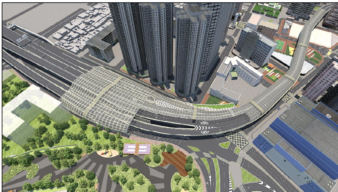
建議緩解噪音設施 - 加士居道天橋 Proposed Noise Mitigation Measures - Gascoigne Road Flyover
