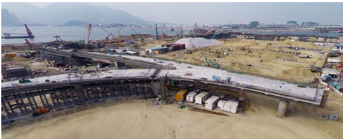
Figure 8: Construction of bridge infrastructures of the HKBCF is in progress.
