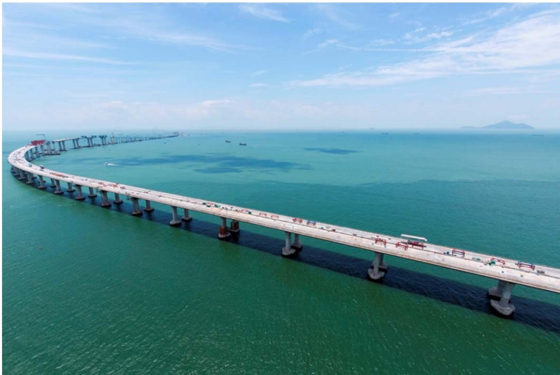
Figure 9: Construction of the marine viaduct of the HKLR is in progress.
