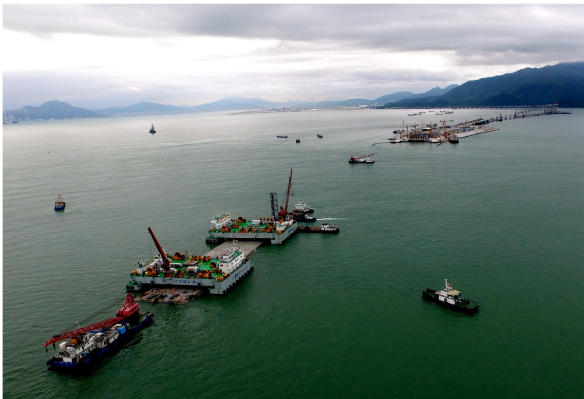
Figure 3: Installation of a tunnel segment of the HZMB Main Bridge.
