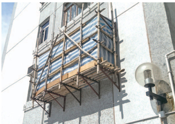
研究針對如何改良 I 型狗臂架的設計，從而提升從業員的高空工作安全。 The research on ways to modify the design of "I" type brackets which supports the truss-out scaffold could effectively improve safety protection for working-at-height.
