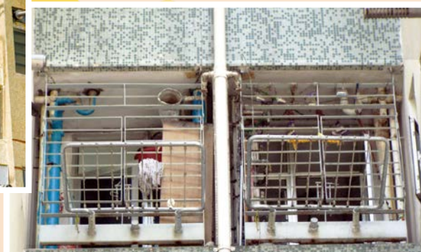
Parallel type laundry racks installed at Chak On Estate (left) and perpendicular ones at Shek Yam East Estate
