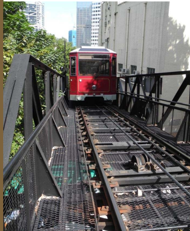
Foundation and Bridge strengthening 鞏固地基及橋樑
