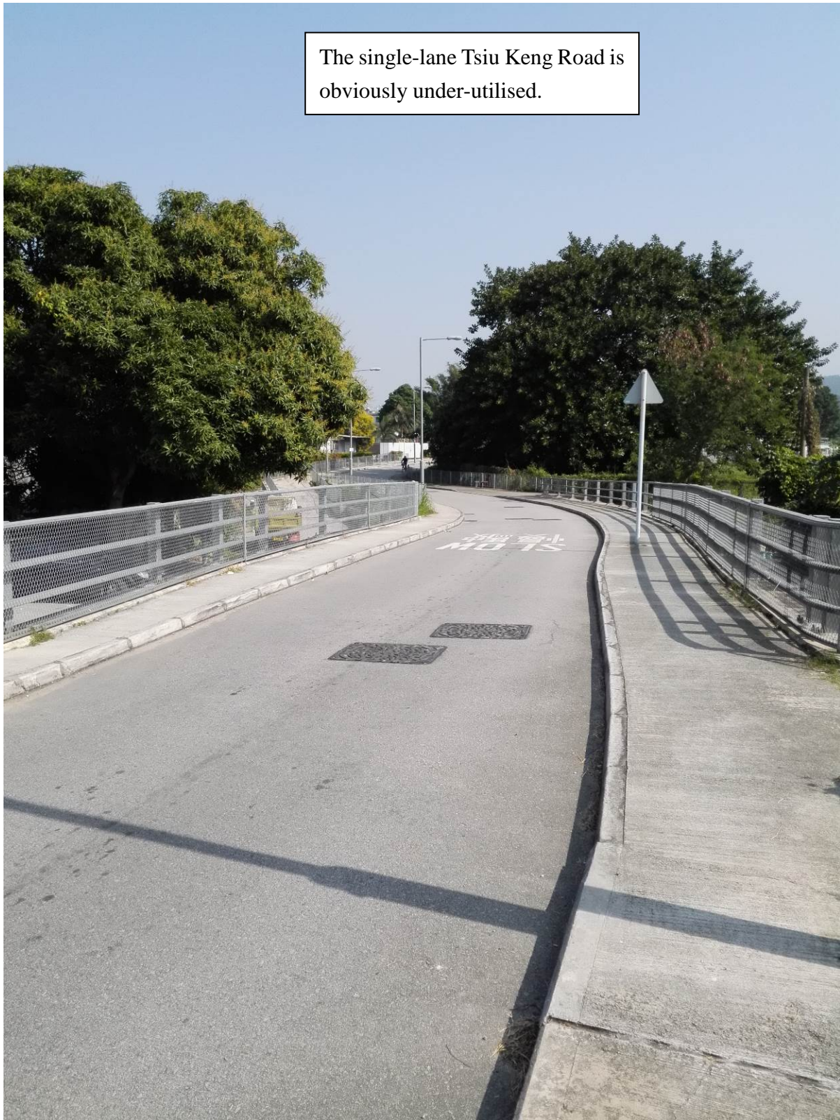
Figure 1. The existing situation of Tsiu Keng Road (photographs taken in December 2017).
