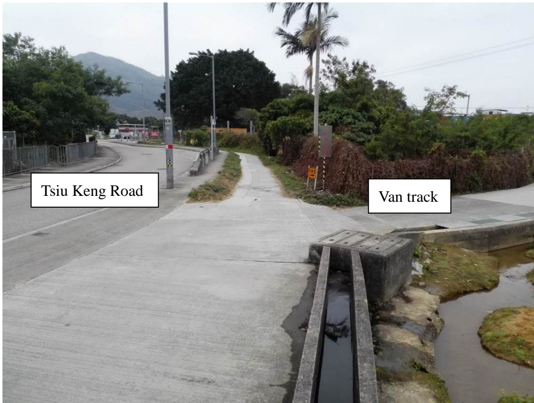
Figure 2. Some van tracks/ footpaths leading off/ extending from the Tsiu Keng Road.
