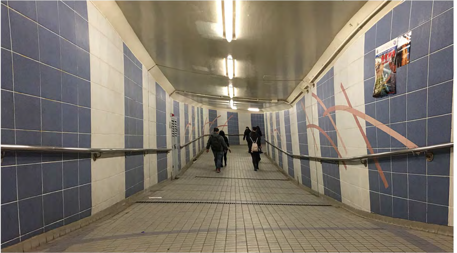
柯士甸道行人隧道內 - 現時狀況 INTERIOR OF AUSTIN ROAD PEDESTRIAN SUBWAY - EXISTING CONDITION
