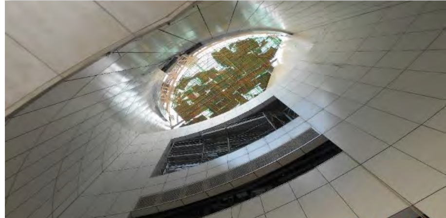
General view for aluminium cladding wall 鋁合金骨架外牆
