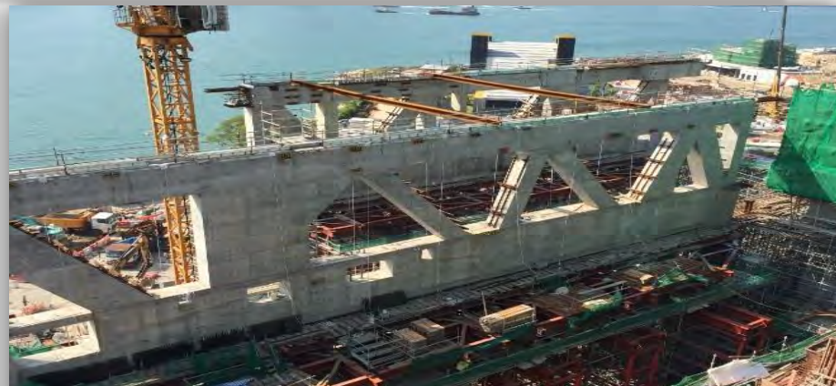
General view for T3 & T4 mega truss T3 和 T4 桁架概覽
