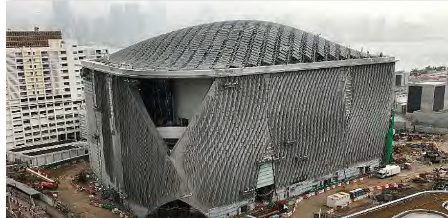
General view for façade with fin installation 外觀及終飾安裝
