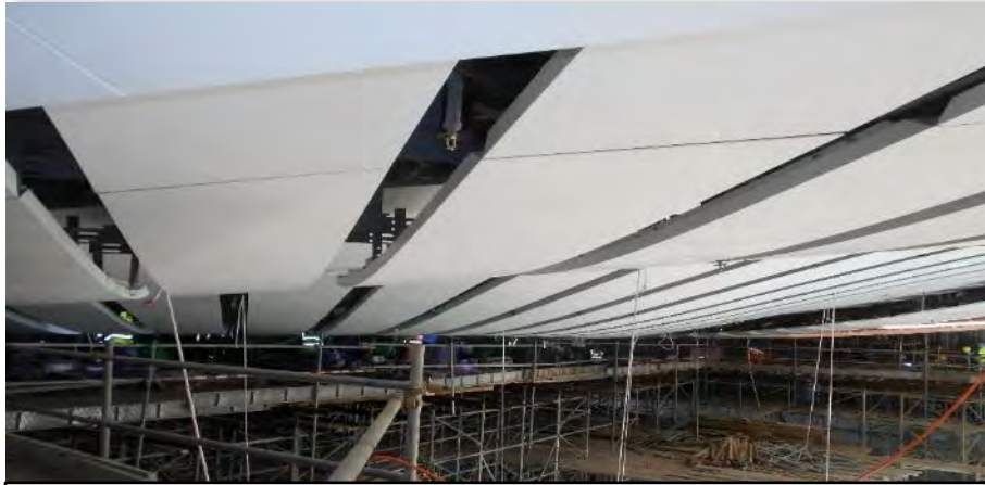
General view for Atrium ceiling installation 中庭天花安裝
