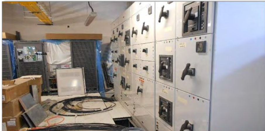
Mechanical, Electrical, Plumbing (MEP) works in progress 機電工程安裝進行中
