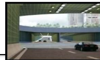
Depressed Austin Road West and Lin Cheung Road junction 低於地面的柯士甸道西與連翔道交匯處
