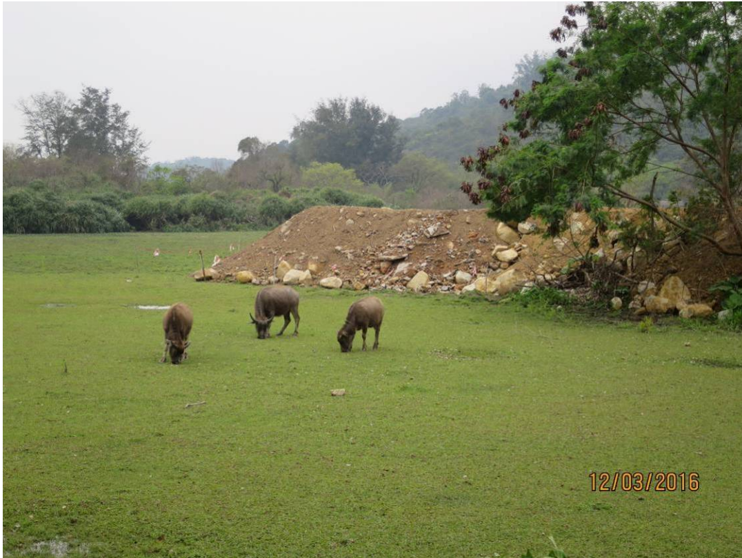
Figure 6. Dumping of rubble and construction waste, concrete paved areas and built structures at the Coastal Protection Area of Pui O.
