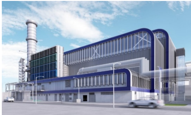
New CCGT Generating Unit D2
