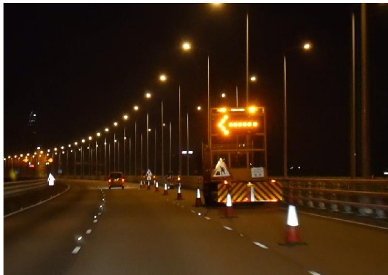
Figure 2 : Provision of shadow vehicle with truck-mounted attenuator and longitudinal safety clearance zone in front of lane closure
