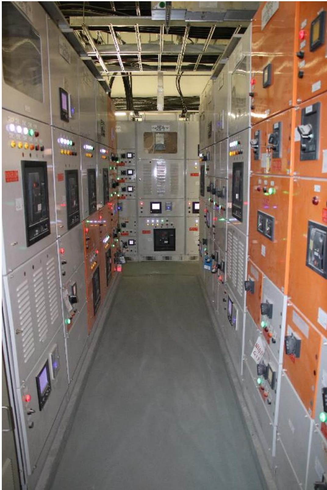
Regarding the water leakage incident at the Passenger Clearance Building of Hong Kong-Zhuhai-Macao Bridge Hong Kong Port, photo (taken on July 3, 2018) shows the present condition of the location of the April 15, 2018 water leakage incident.
