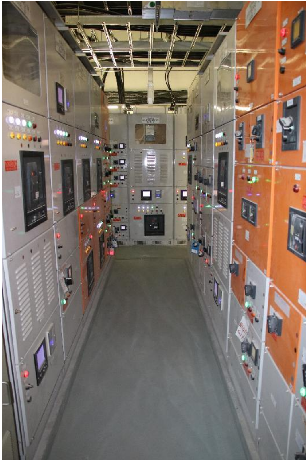
Regarding the water leakage incident at the Passenger Clearance Building of Hong Kong-Zhuhai-Macao Bridge Hong Kong Port, photo (taken on July 3, 2018) shows the present condition of the location of the April 15, 2018 water leakage incident.
