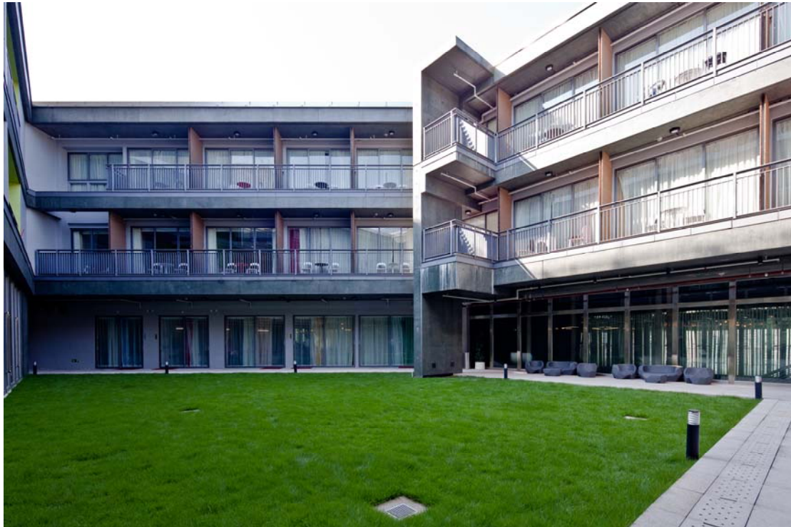
Y-Loft (Main Block)
