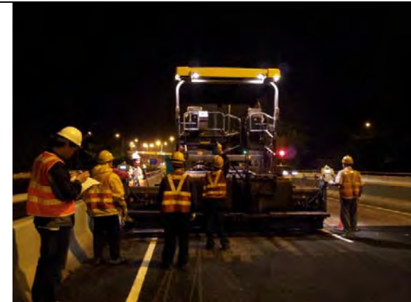
Road paver paving the layer
